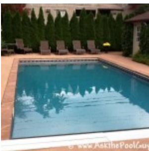
Coping Stone Slabs
